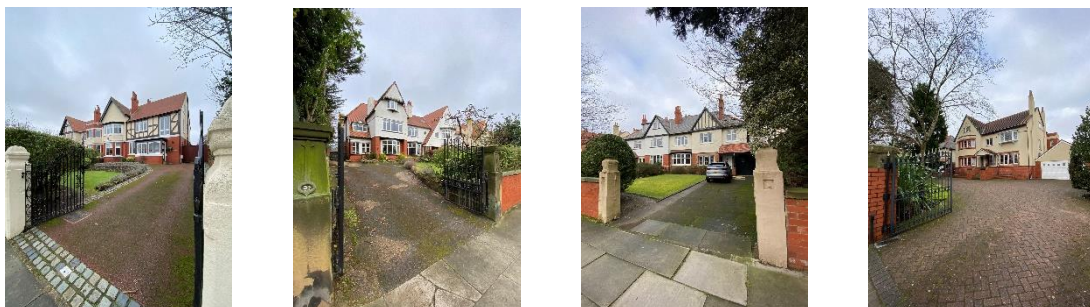
From left to right, Nos. 36, 32, 24 and 22 Hesketh Road showing the brick base at ground floor levels.
