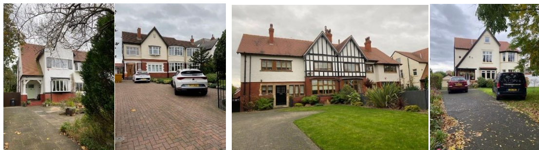
From left to right; No. 20, No. 16, Nos. 6-8 and No.4 Argyle Road.
