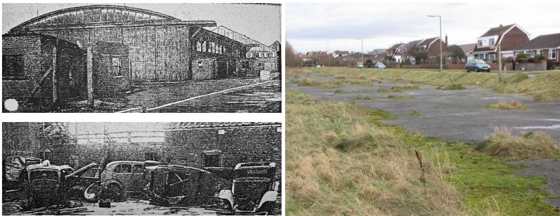
Photograph of the hangars in 1965 used to dump old cars. Remains of the apron are still visible today on site.
