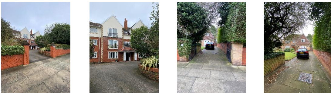
From left to right, No. 12 Hesketh Road, No. 10a Hesketh Road
